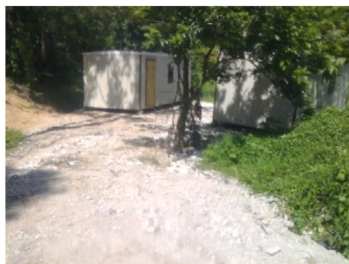
Placement of the cabin for the Eco Melawati RCEC
